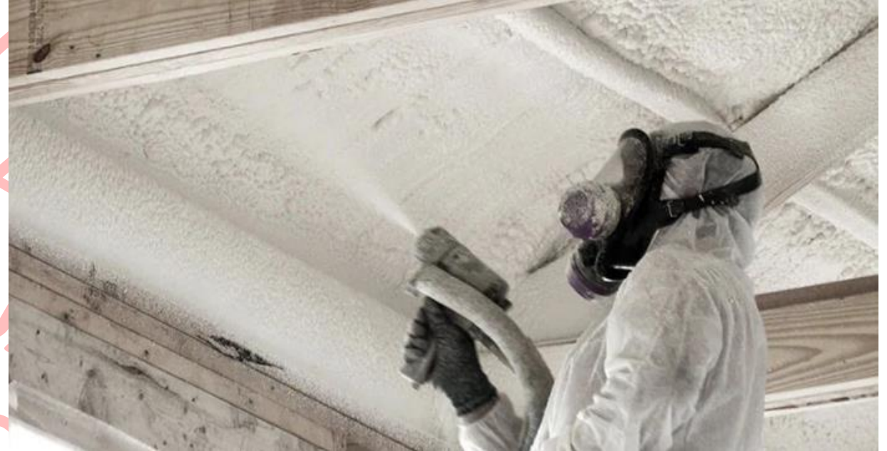
Insulation Foam Spray
